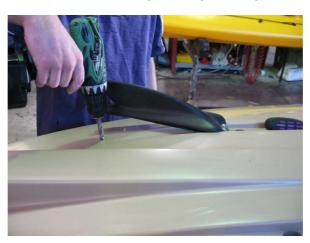
**Step 6:** Remove skeg, and drill rear hole (first with pilot bit, then with 9.5mm drill bit). Insert well nut into rear hole. Before final attachment of skegs, it is recommended that a marine grade silicone sealant is used in and around the well nuts.
